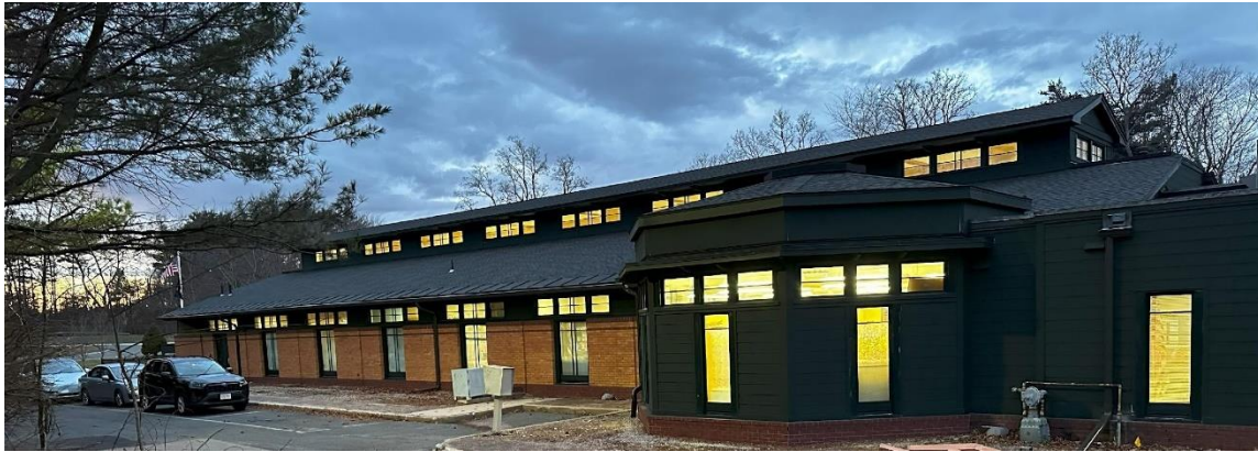
Staff parking and rear entryway; note lack of outdoor overhead lighting
