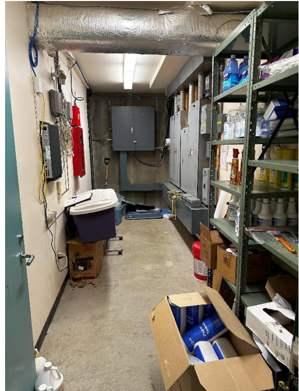
Basement storage area; note electrical and HVAC mechanical systems in space
